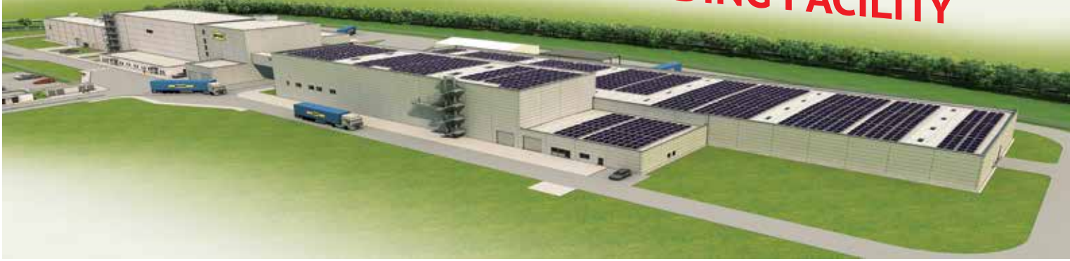
New blending facility in Nettetal
